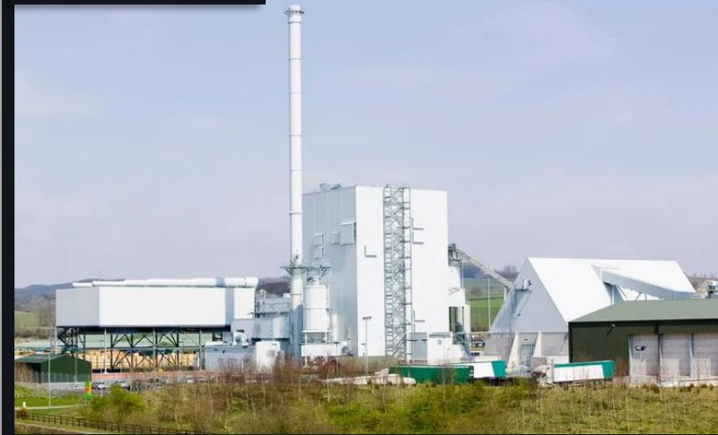
E.ON's biomass power plant near Lockerbie, Scotland, where the e-methanol project will be built. (Photo: Construction Photography/Avalon/Getty)
